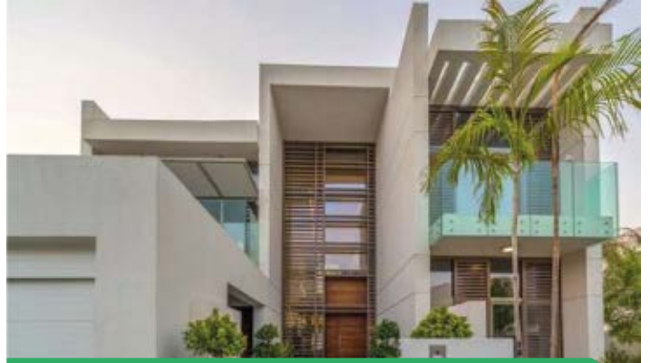
Project: Dohler Middle East factory, Jebel Ali, Dubai Project: Private villa at Mohammed Bin Rashid City – District One Scope of work: Revamp & Preventive Maintenance Service Brand: Daikin Type of Machines: VRF System, Home automation system
